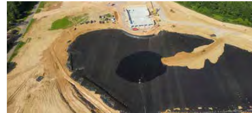
Digging man-made lake
